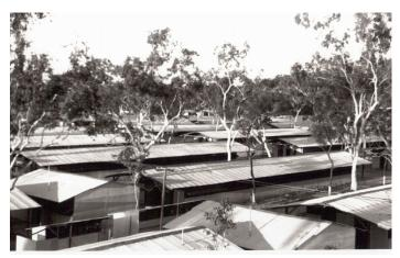
Prefabricated tents were insulated and included adjustable shutters, a wooden floor and a corrugated iron roof.
