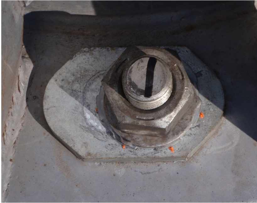
Figure 18 – View of an installed plate washer
