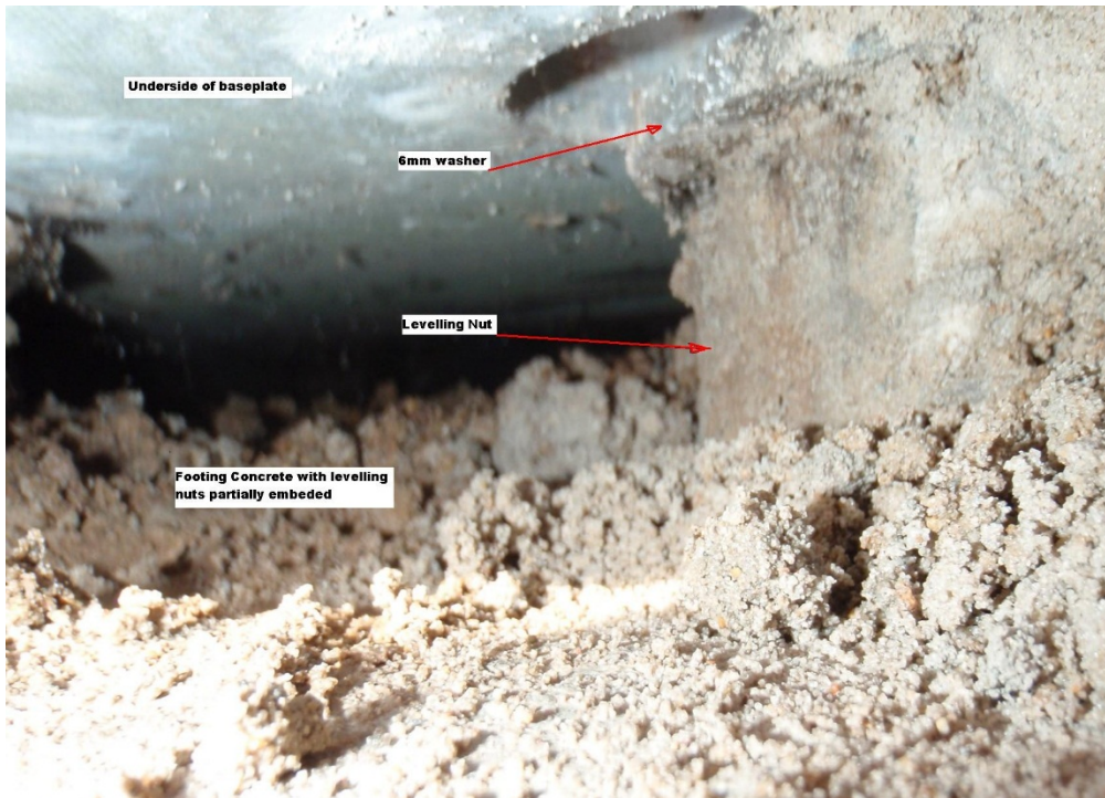
Figure 3 – View under the base plate
