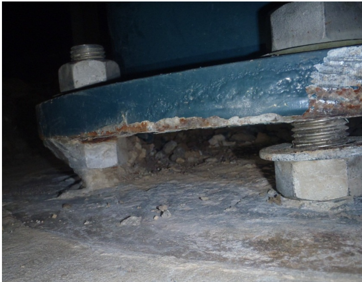
Figure 13 – View of the mortar removed from under the gantry
