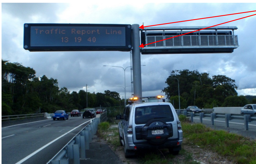
Figure 19 – View of the splice joint location
