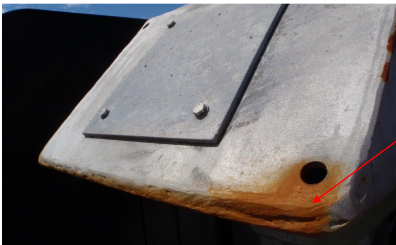
Figure 38 – Corrosion leaching out of vent hole
