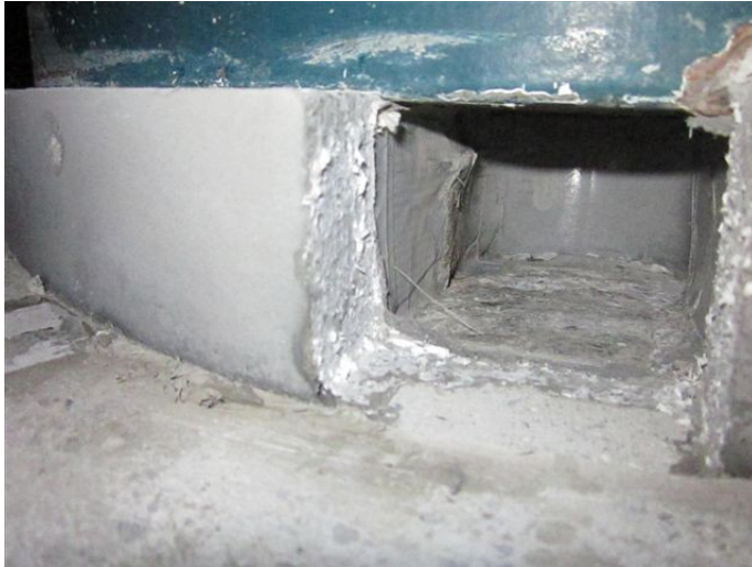
Figure 12 – View of the pocket created by the removed wedge
