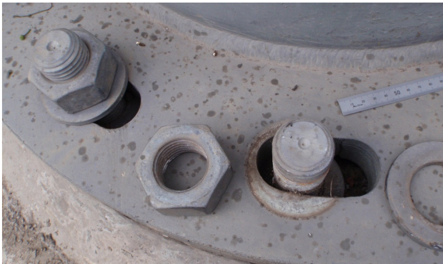
Figure 5 – Hold down nut was loose
