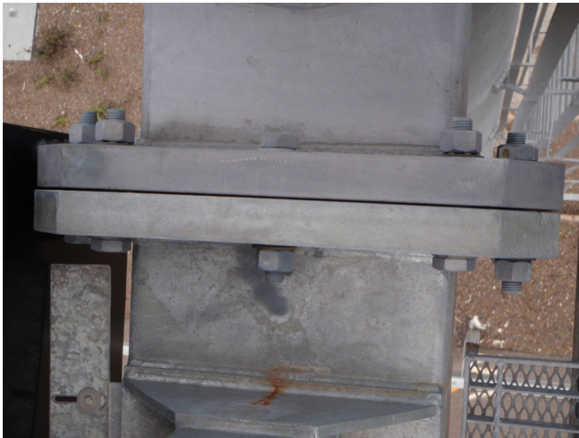
Figure 21 – Splice joint not pulled together
