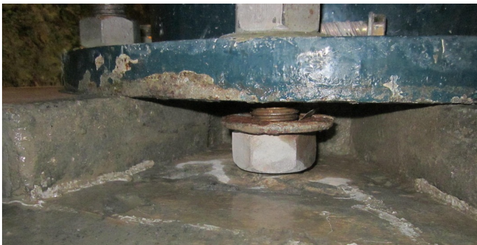
Figure 15 – View of the mortar and installed wedge
