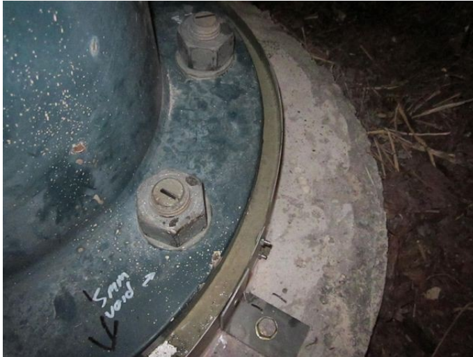
Figure 10 – View of the formwork placed around the footing
