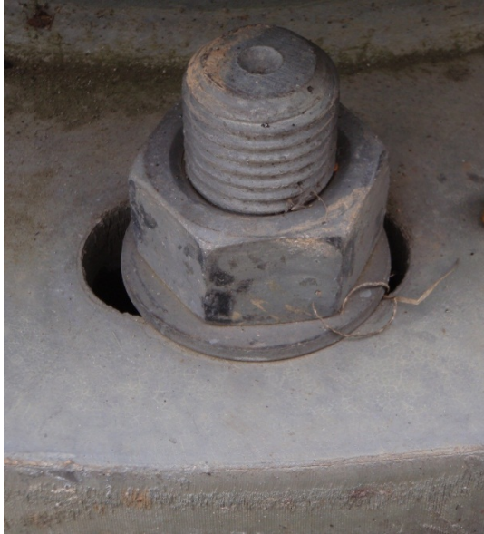
Figure 5 – Hold down nut was loose
