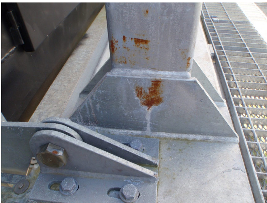
Figure 41 – Corrosion from the vent hole
