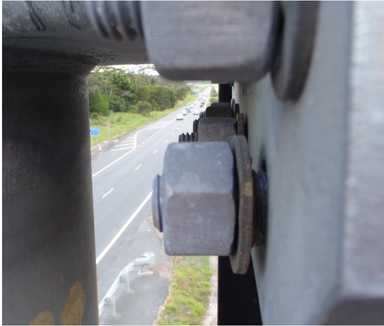
Figure 21 – Splice joint not pulled together
