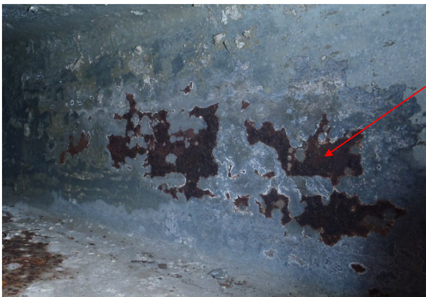
Figure 41 – Corrosion from the vent hole
