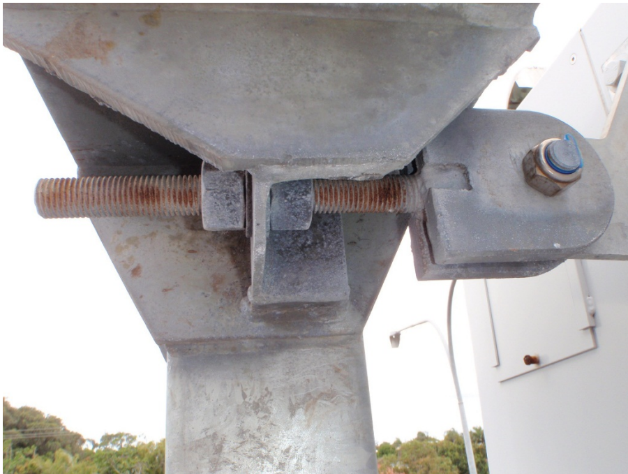
Figure 43 – General corrosion on the threads
