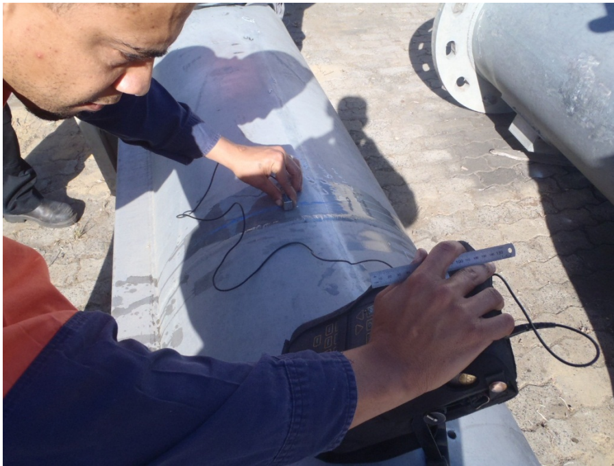
Figure 49 – View of the method of testing the welds
