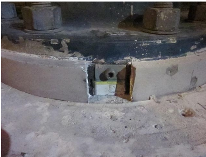
Figure 11 – View of the mortar and installed wedge
