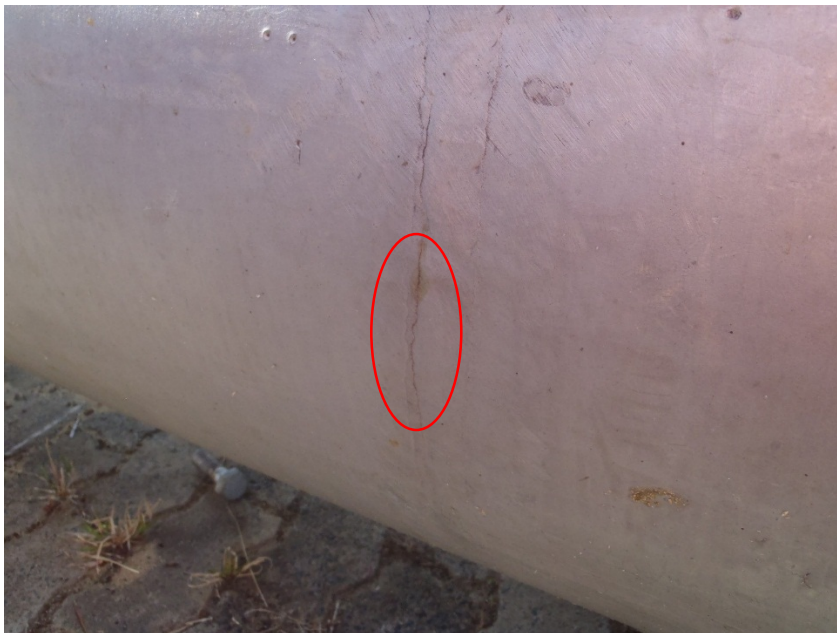
Figure 48 – View of the visual cracks in the butt weld on the back side of the column member
