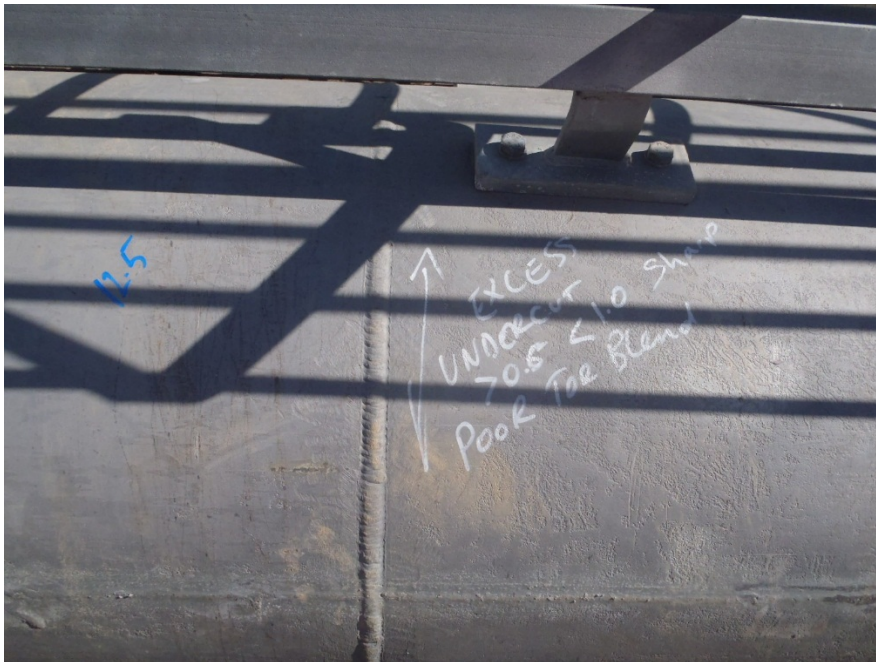
Figure 52 – View of the level of undercut in the butt weld
