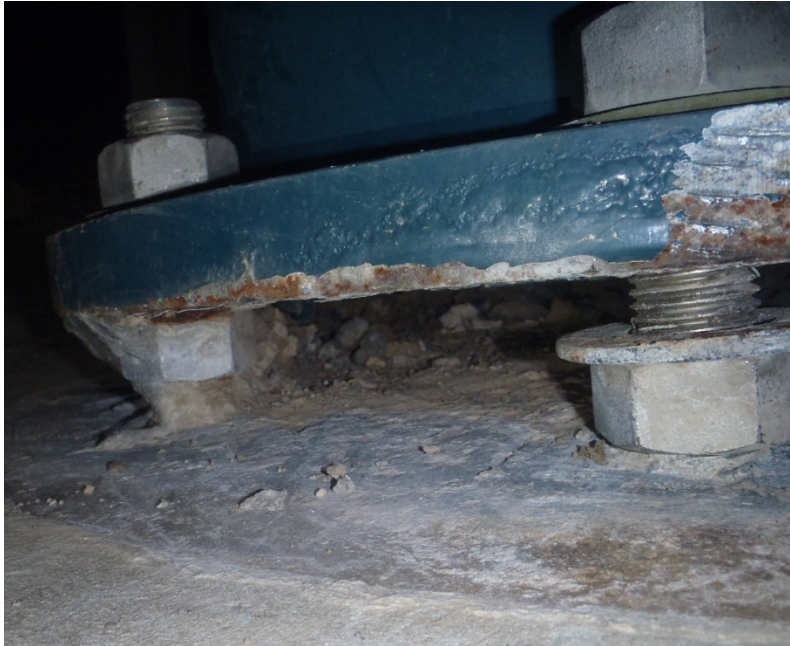
Figure 9 – View of the mortar removed from under the gantry
