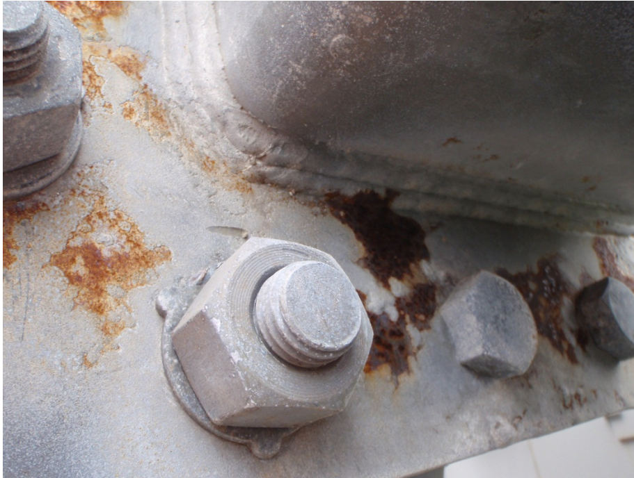
Figure 43 – General corrosion on the threads
