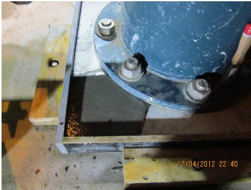
Figure 16 – View of the pocket created by the removed wedge
