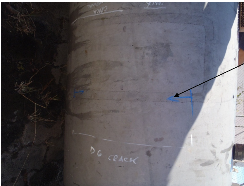
Figure 50 – View of the marked out area
