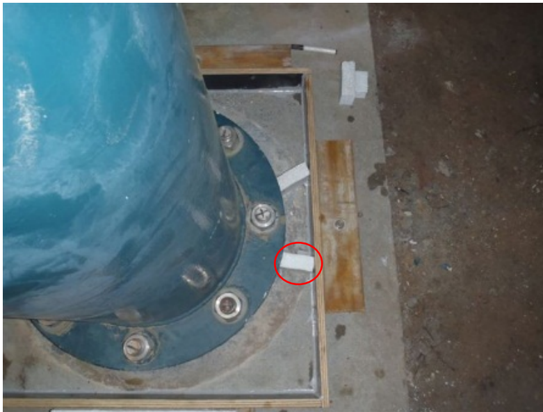
Figure 14 – View of the foam around the levelling nut
