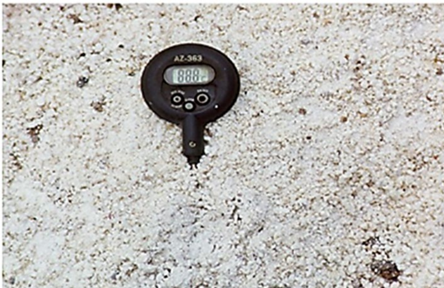
Figure 8.6.6.2.3 – Checking completion of slaking with temperature probe
