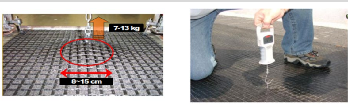
Figure 10.2.5 – Spring balance test to measure the construction bond strength
