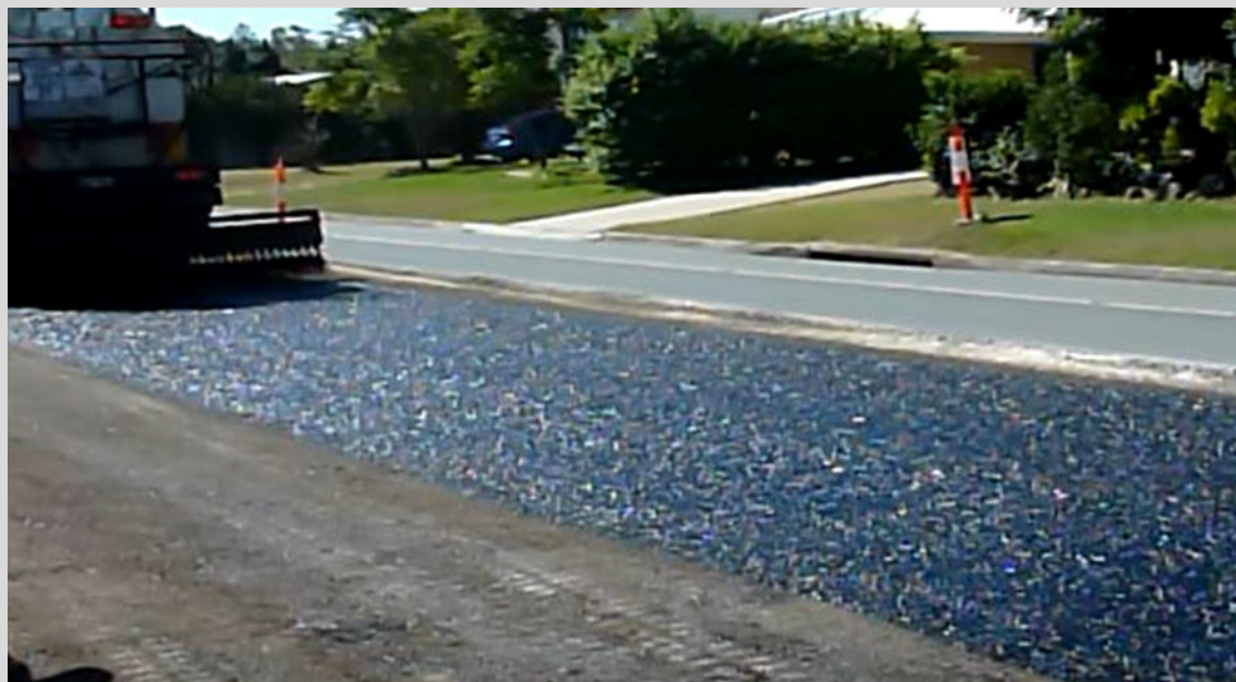
Figure 9.5.3 – Example of C170 bitumen bond coat sprayed on a prepared pavement surface
