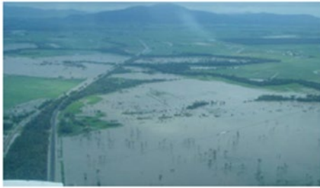
Figure 4.8.2 – Murray River Crossing of Bruce Highway
