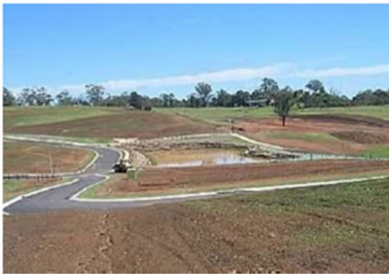
Figure 1.6.2 – Detention basin in a residential subdivision
