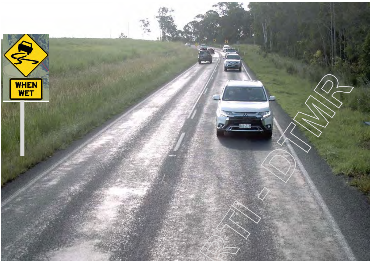
Tdist 5.32km RHS AG – Install W5-20B and W8-7B Slippery when wet warning signs
