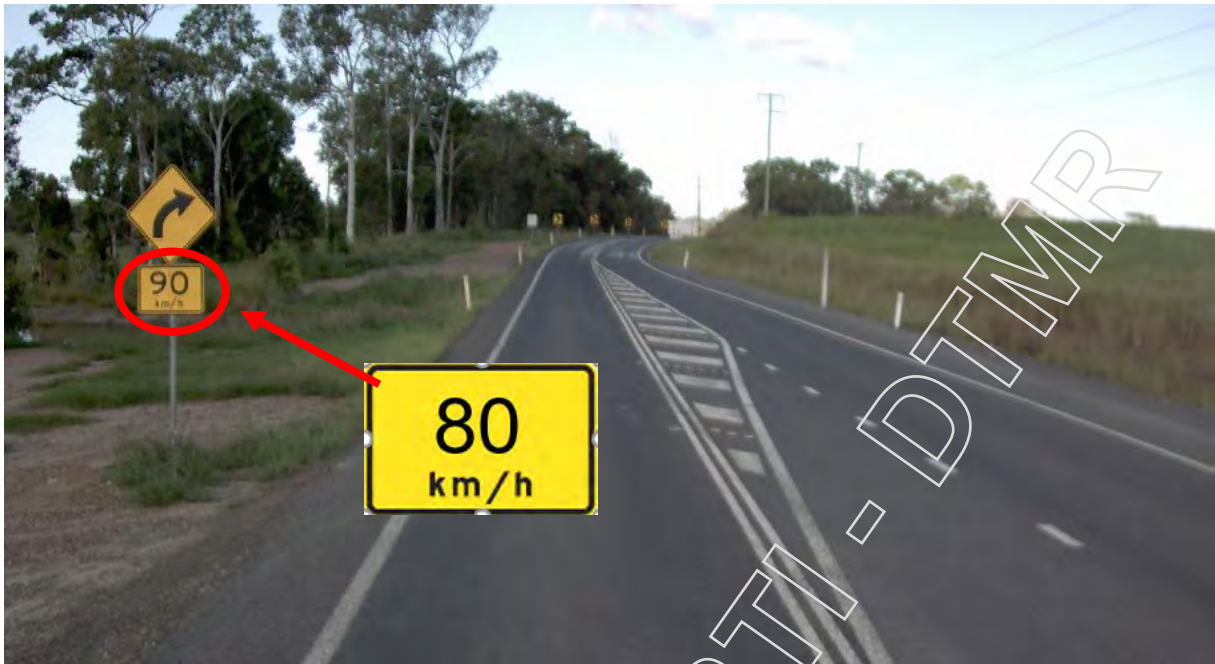
Tdist 4.86km LHS WG – Replace existing 90km/h advisory speed plate with 80km/h advisory speed plate (W8-2B)
