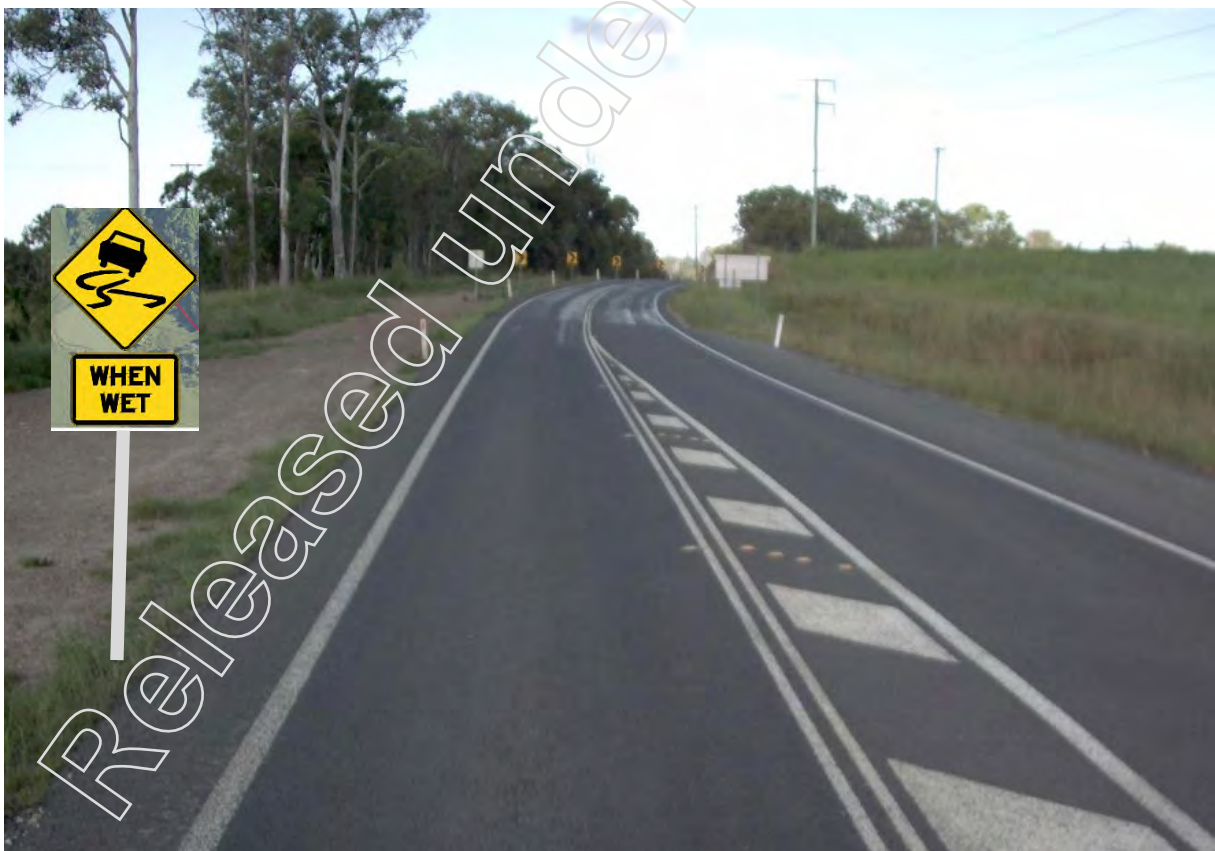
Tdist 4.92km LHS WG – Install W5-20B and W8-7B Slippery when wet warning signs
