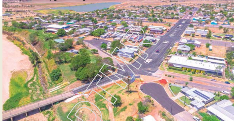
Gray Street upgrade Hughenden.
