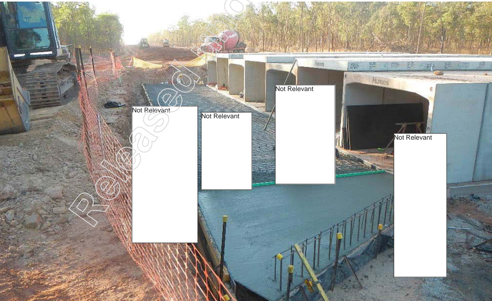
Installing culverts at the Kennedy to Rocky Creek project, Peninsula Developmental Road, Cape York Region Package.
