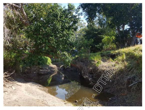
Figure 8 Scour hole looking upstream towards Rail Bridge
