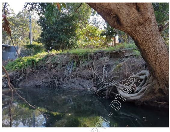
Figure 10 Collapsed banks
