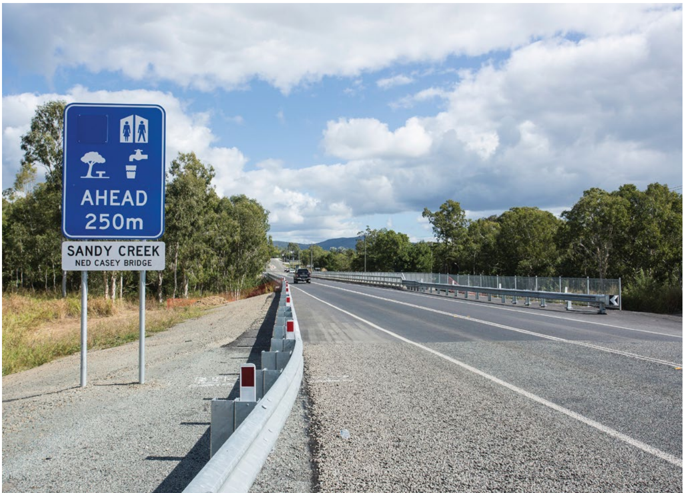
Ned Casey Bridge, Sandy Creek, Eton
