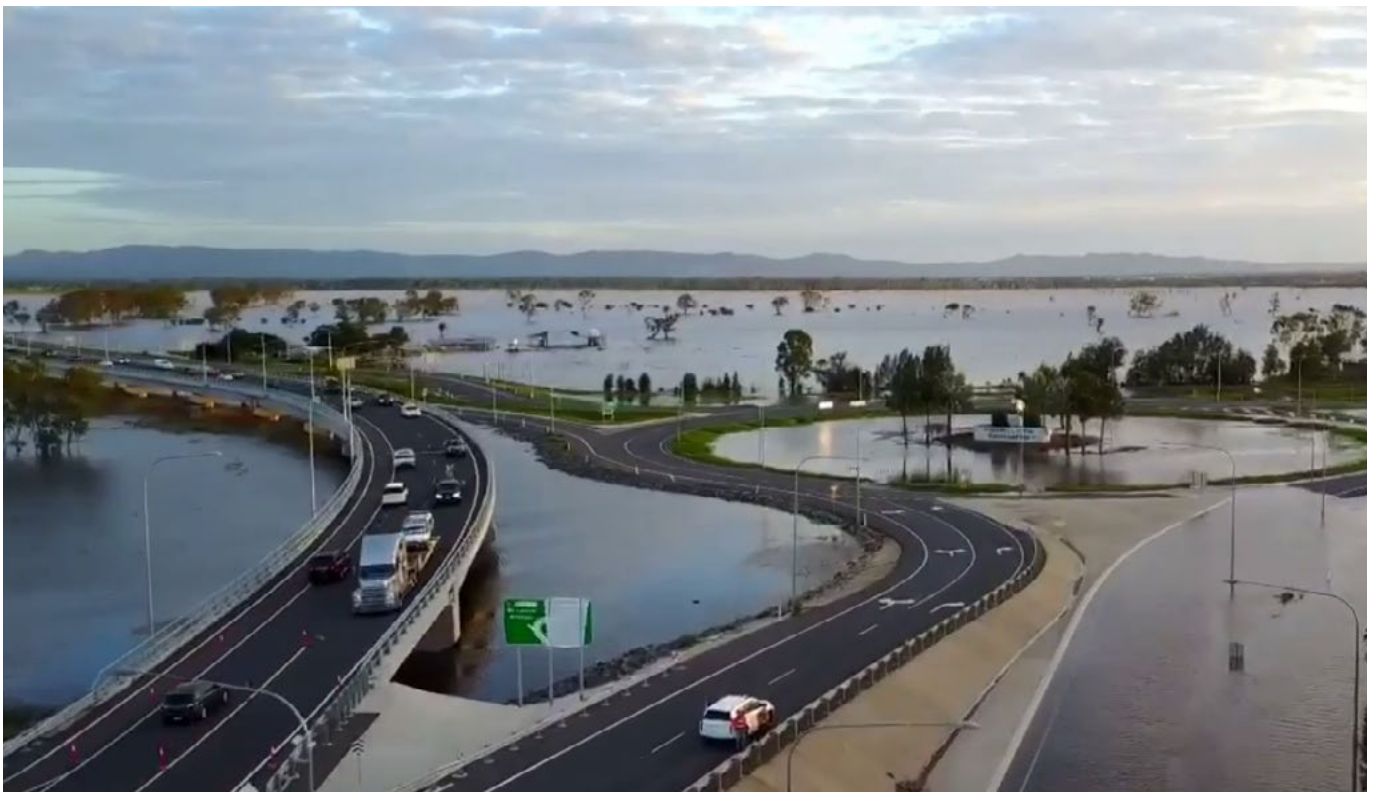
Yeppen Floodplain bridges, Rockhampton
