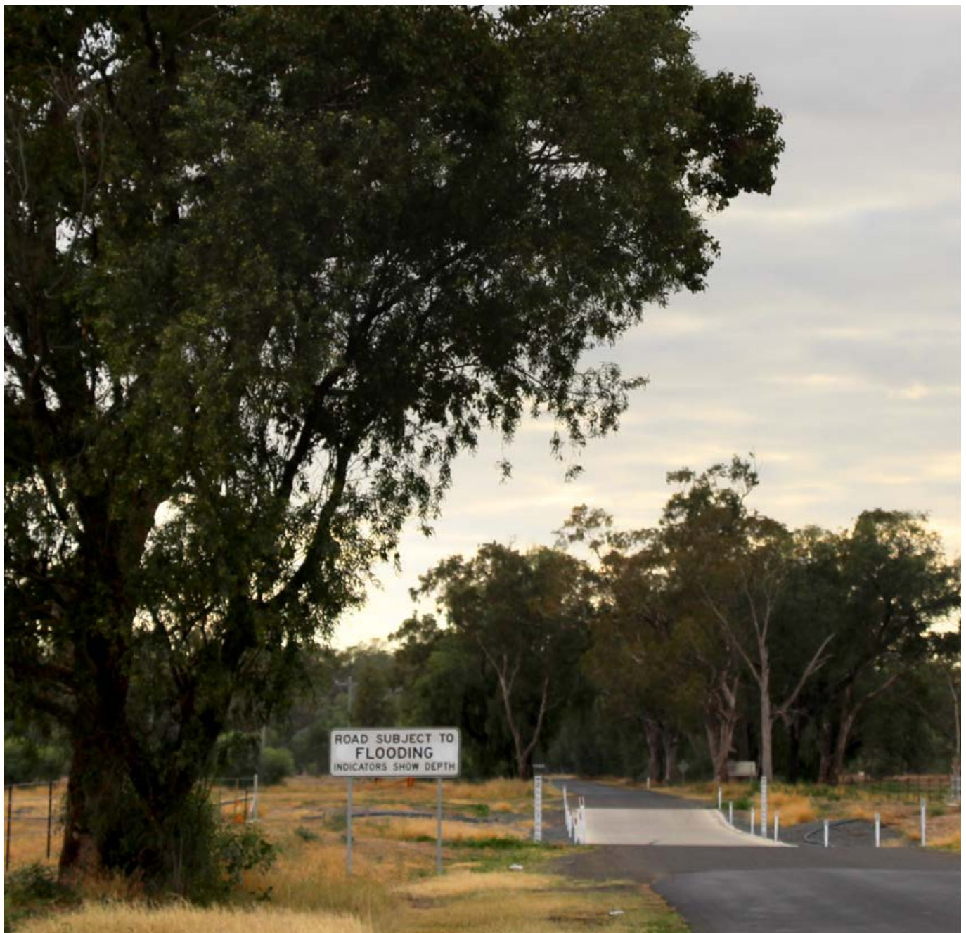
Flood warning sign, Ashburn Road, Roma
