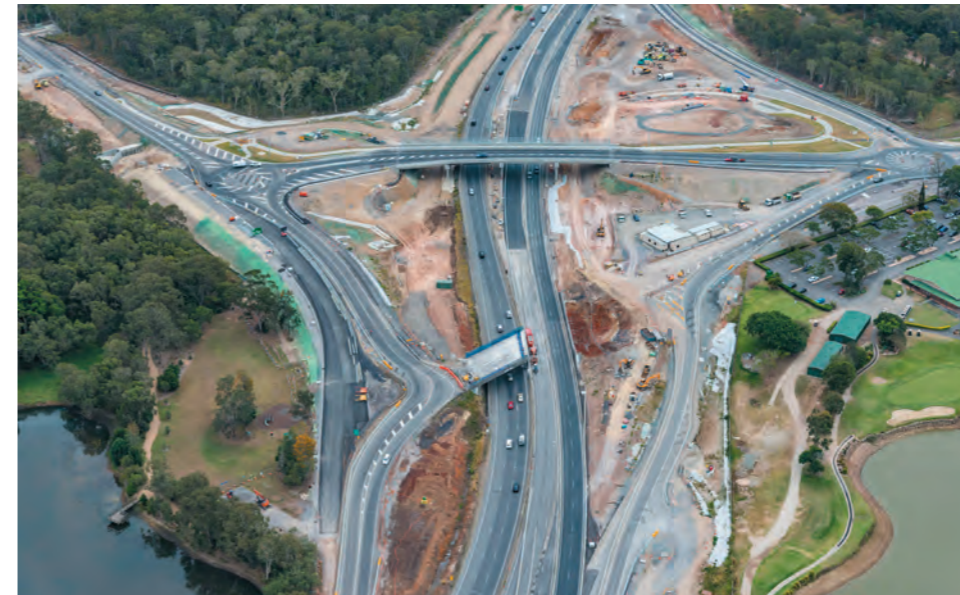
Upgrade of Nudgee Road interchange (looking north)
