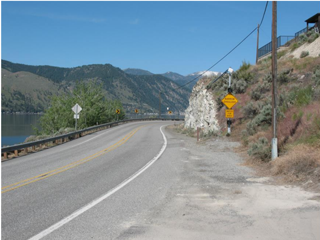
Figure 8(b) – Narrow roadway (no shoulder), Rocky Point, Washington USA
