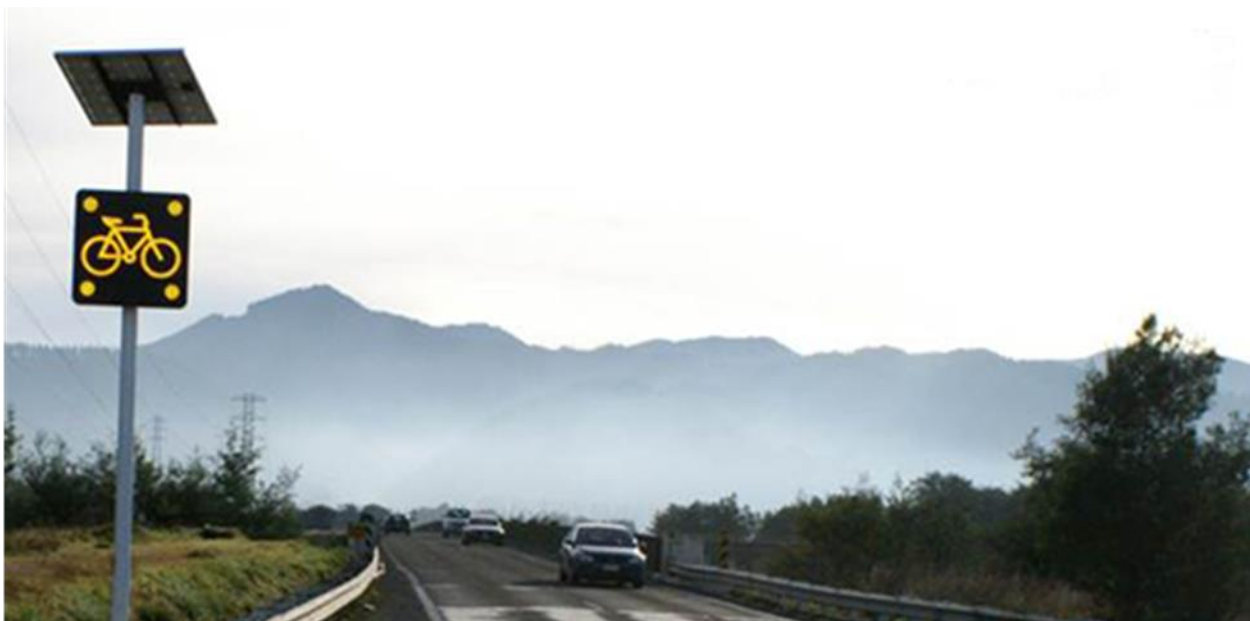
Figure 8(a) – Narrow bridge treatments in Marlborough and Arthur, New Zealand
