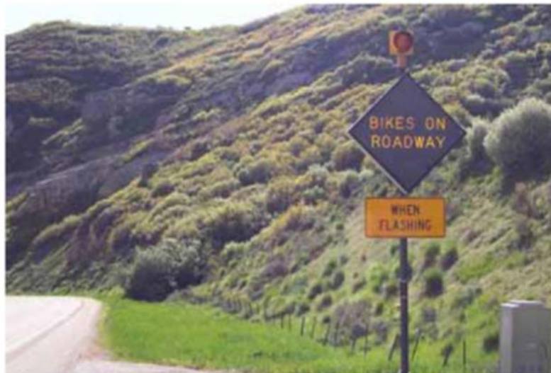
Figure 6(c) – Active warning sign on a narrow winding road near Steamboat, Colorado
