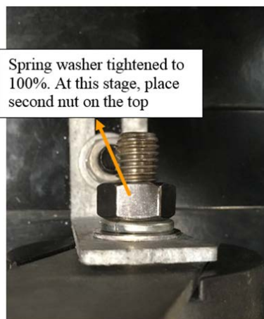
Figure 4.3(c) - Spring washer fully tightened
