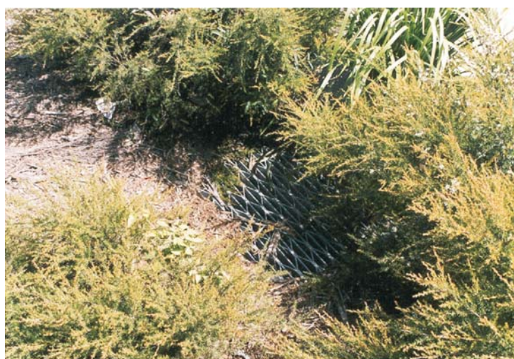
Figure 6.11 Surface view of a culvert skylight
