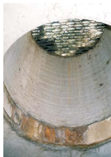
Figure 6.12 View of skylight in roof of culvert
