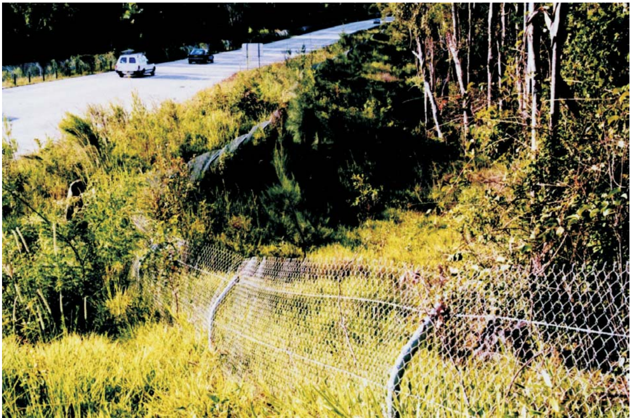
Figure 6.17 'Floppy-top' fencing designed to prevent Koalas entering the road reserve (Brunswick Heads Bypass, northern NSW)
