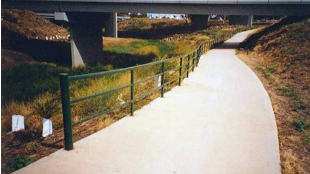
Figure A14 – Cyclist travelling downhill has positioned himself on the centre of the path away from the fence, which remains a snag hazard for children
