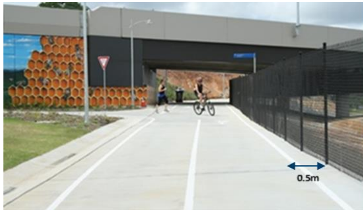
Richlands Railway Station Precinct Source: Fullframe Photographics
