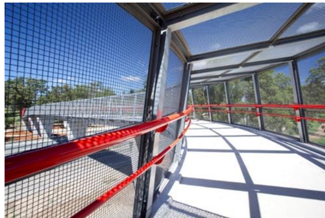
Figure A11 – Photo showing separate hand rails for pedestrians and cyclists
