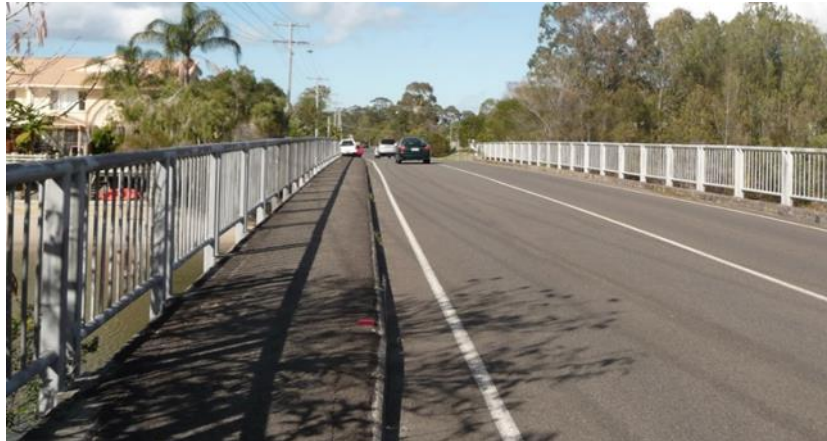
Figure A10 – Photo showing path used by cyclists with a kerb separation to traffic lane
