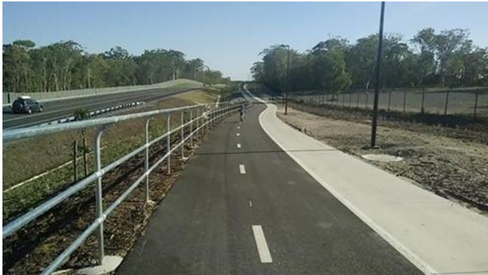
Figure A14 – Cyclist travelling downhill has positioned himself on the centre of the path away from the fence, which remains a snag hazard for children
