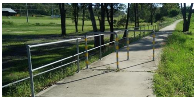
Figure A1 – The fence on the path may pose a greater risk to users than other hazards
